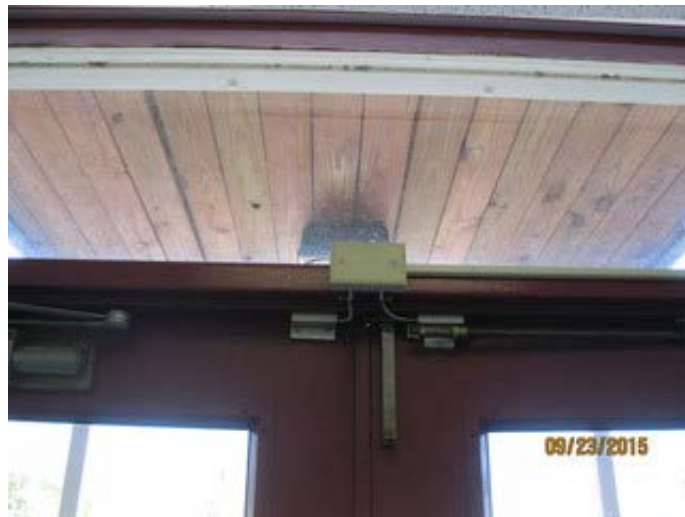
Door Contacts for Security System
