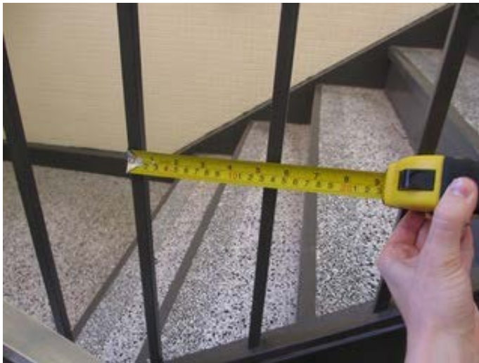
Guard rails do not meet the 4 inch ball test
