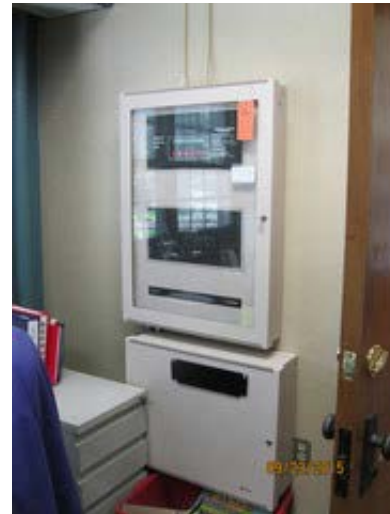
Fire Alarm Control Panel
