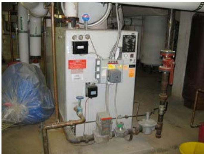
Gas Fired Boiler
