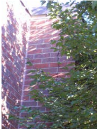
Crack in Wall
