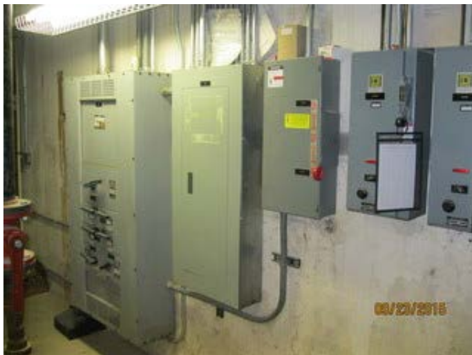
Electrical Panels in Boiler Room
