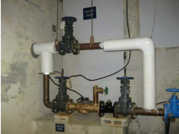
Main Water Service With Meter
