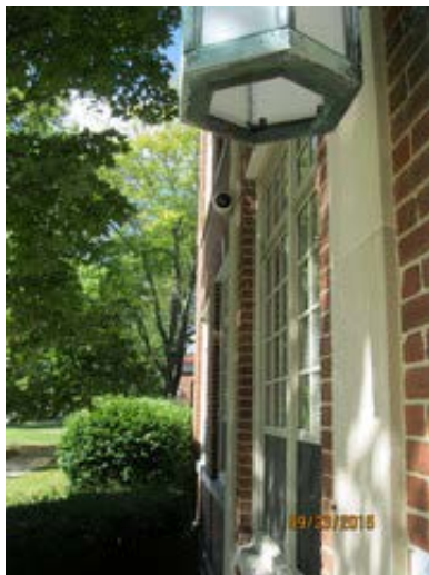
Access Control Camera at Main Door
