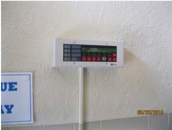
Fire Alarm Remote Annunciator
